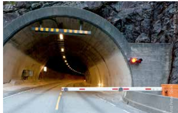
Closing of tunnels with barriers.
